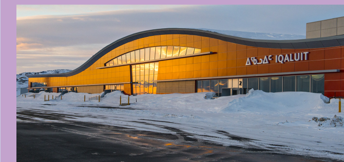
IQUALUIT AIRPORT We fabricated and erected the new terminal building and Fire services hangar of the Iqaluit International Airport that serves Iqaluit, the only city in the northern territory of Nunavut, Canada.
