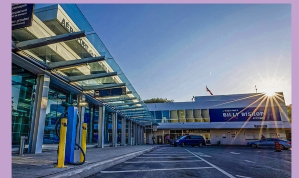
BILLY BISHOP AIRPORT, Benson fabricated the structural steel for this airport that welcomes 2.8 million travelers each year. It is Canada's sixth-busiest airport that offers passenger service to the United States. Billy Bishop Airport is renowned for its unique travel experience, efficiency and customer service.
