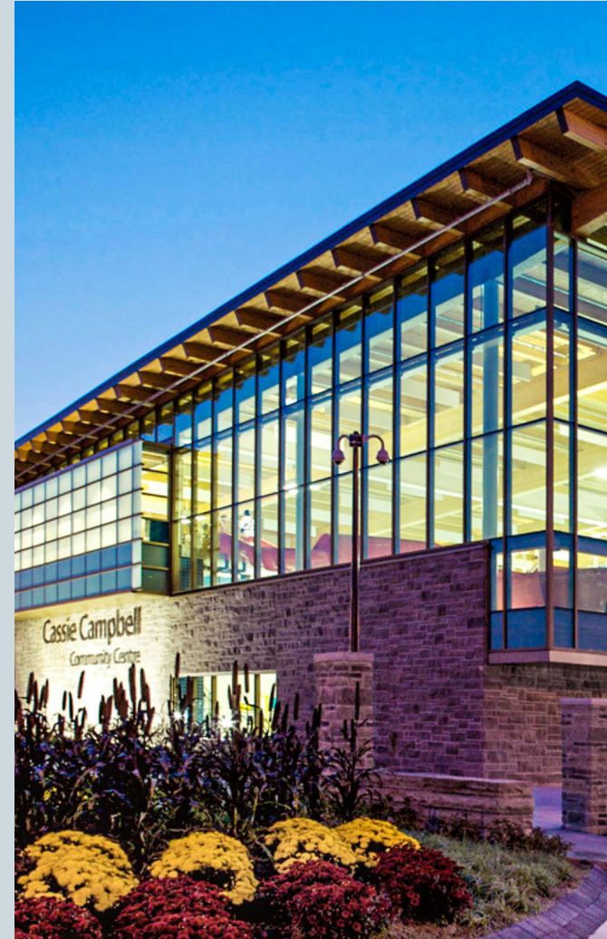
CASSIE CAMPBELL COMMUNITY CENTRE Bramton, Ontario, Canada
