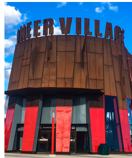
TTC TRANSIT STATION Pioneer Village Toronto, Ontario, Canada
