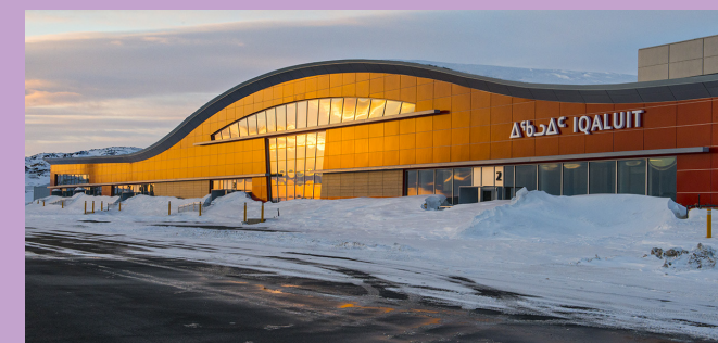
IQUALUIT AIRPORT We fabricated and erected the new terminal building and Fire services hangar of the Iqaluit International Airport that serves Iqaluit, the only city in the northern territory of Nunavut, Canada.
