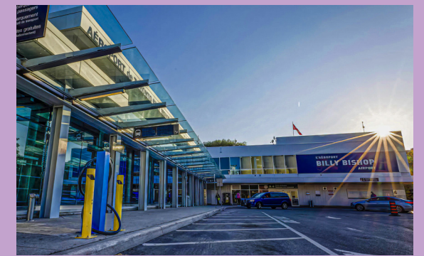
BILLY BISHOP AIRPORT, Benson fabricated the structural steel for this airport that welcomes 2.8 million travelers each year. It is Canada's sixth-busiest airport that offers passenger service to the United States. Billy Bishop Airport is renowned for its unique travel experience, efficiency and customer service.
